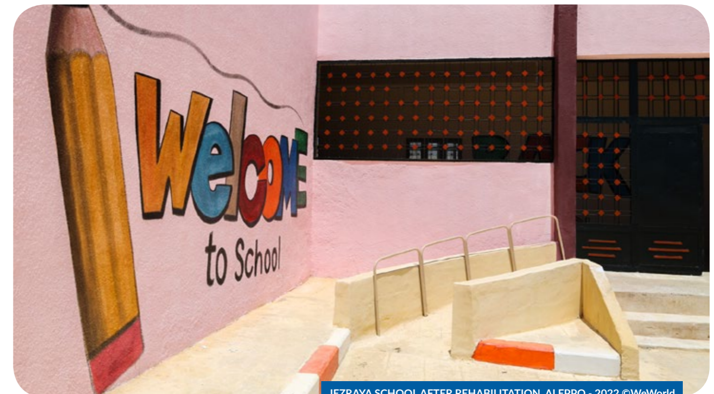
JEZRAYA SCHOOL AFTER REHABILITATION, ALEPPO - 2022 ©WeWorld
